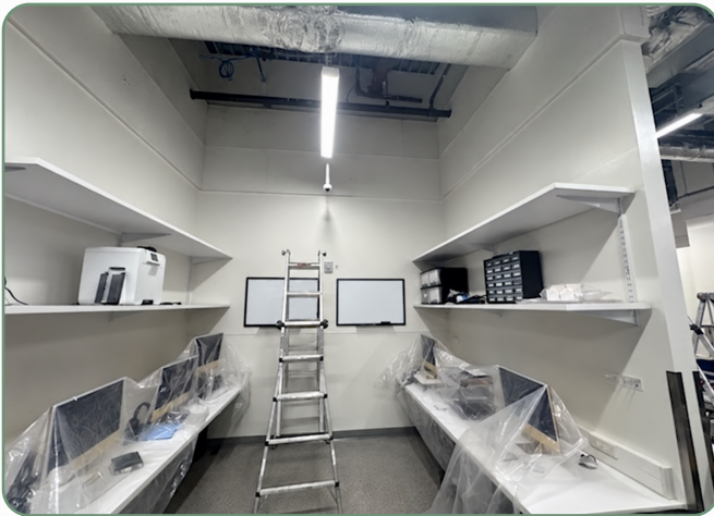
ELECTRONICS PROTECTION | IN PROGRESS
