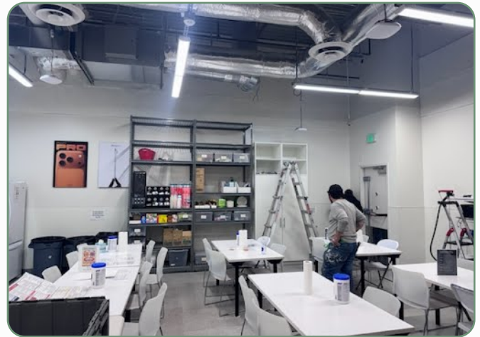
STAFF-AREA PAINTING | IN PROGRESS
