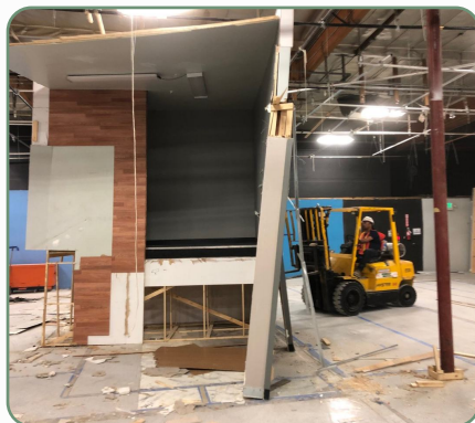
FORKLIFT-ASSISTED SET REMOVAL
