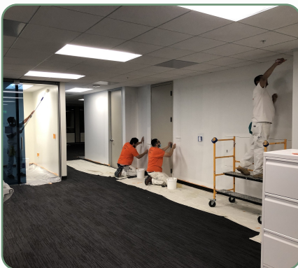
PAINTING CREWS | IN PROGRESS
