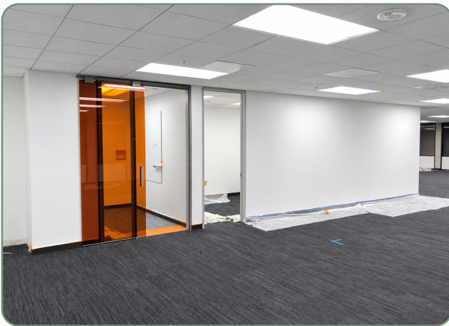
INTERIOR RENEWAL | IN PROGRESS
