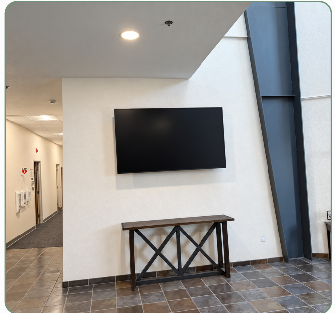
LOBBY DISPLAY INFRASTRUCTURE
