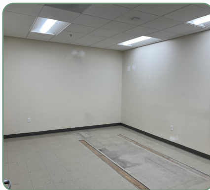
TECHNOLOGY REMOVAL | COMPLETED
