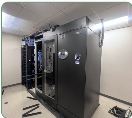
TECHNOLOGY INFRASTRUCTURE | BEFORE
