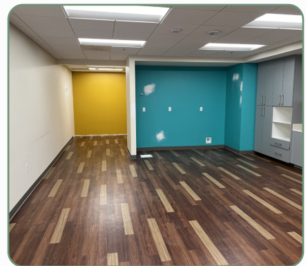
BREAKROOM DECOMMISSION | COMPLETED
