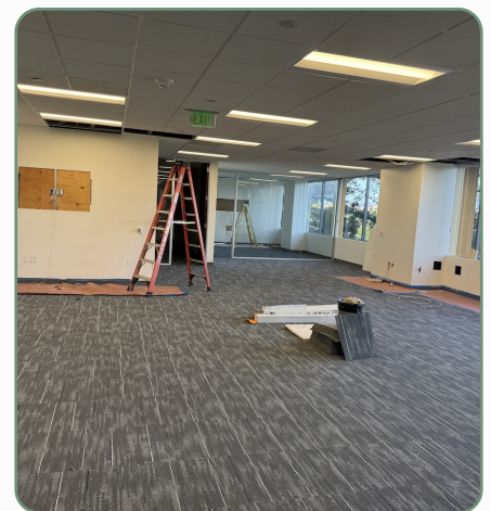
WORKPLACE PREPARATION | IN PROGRESS
