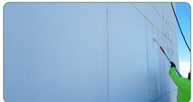
CERTIFIED EXTERIOR ACCESS AND FACADE REPAIR
