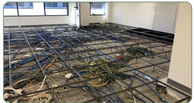
RAISED-FLOOR INFRASTRUCTURE DISMANTLED
