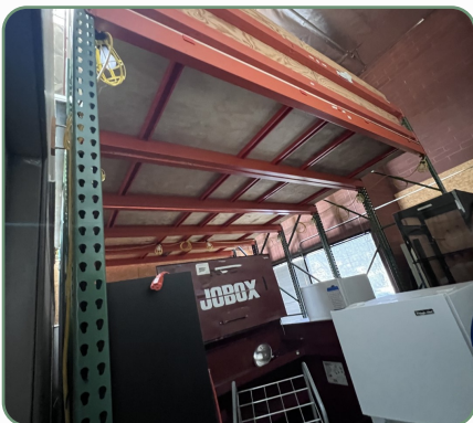
RACK-BUILT MEZZANINE | BEFORE
