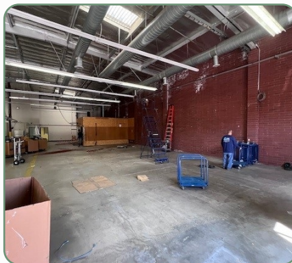
WAREHOUSE CLEARANCE | IN PROGRESS
