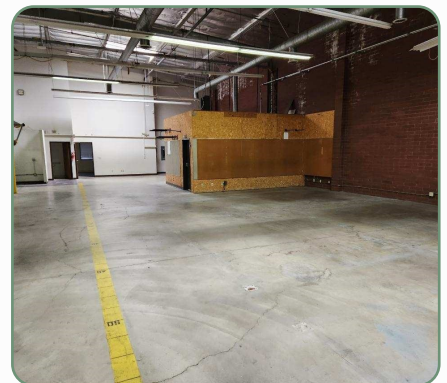
CLEARED WAREHOUSE FLOOR | COMPLETED
