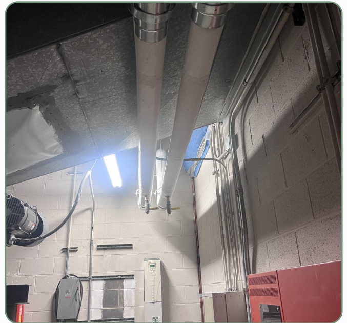
CHILLED-WATER ROUTE | PRE-REMOVAL
