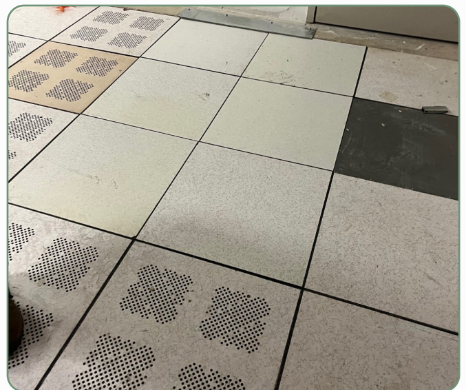
RAISED-FLOOR INFILL | COMPLETED
