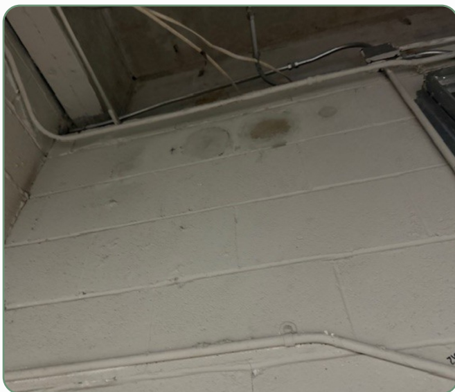
PIPE-ROUTE REPAIR | IN PROGRESS
