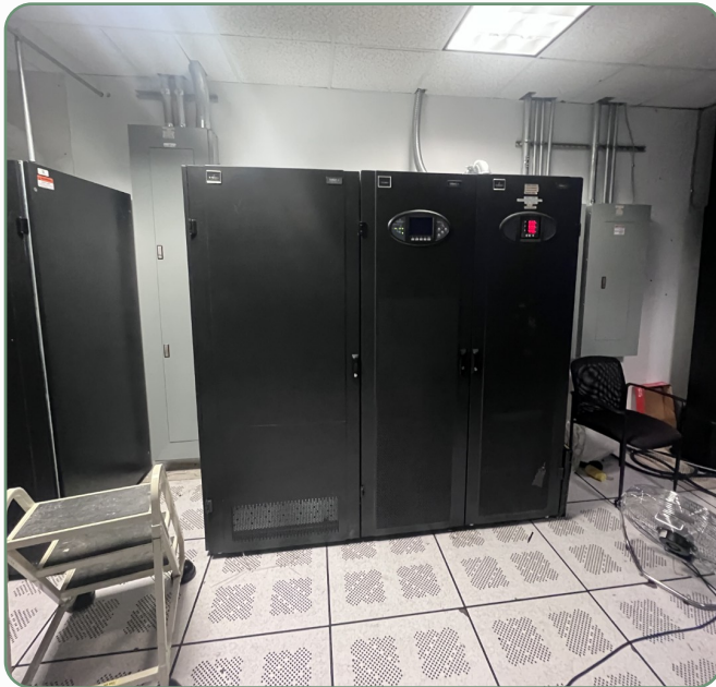
COOLING EQUIPMENT | PRE-REMOVAL
