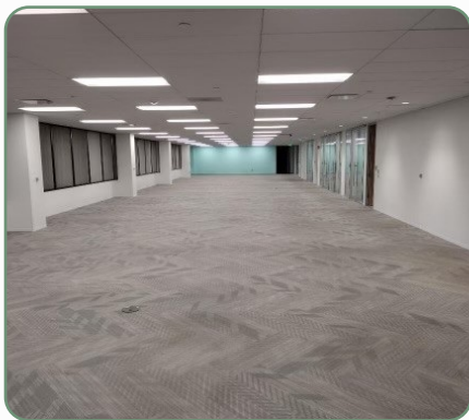
CLEARED OFFICE FLOOR | COMPLETED
