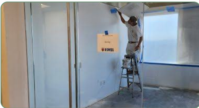
GLENDALE FINISHES | IN PROGRESS
