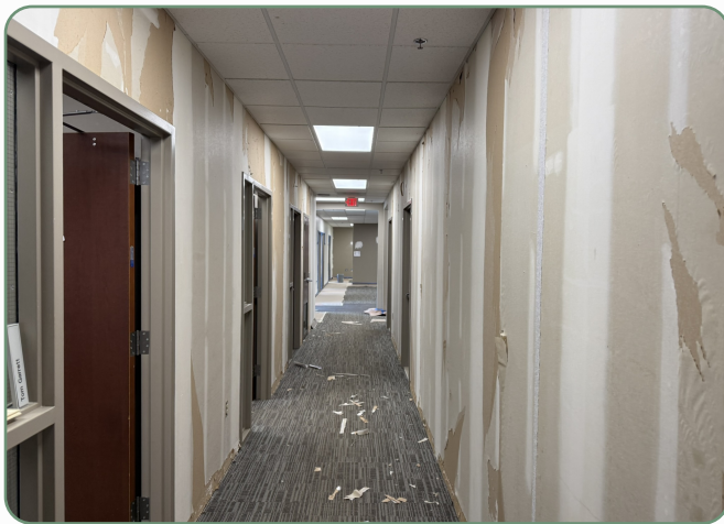
WALLCOVERING REMOVAL | IN PROGRESS
