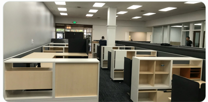
SANTA BARBARA INSTALLATION IN PROGRESS
