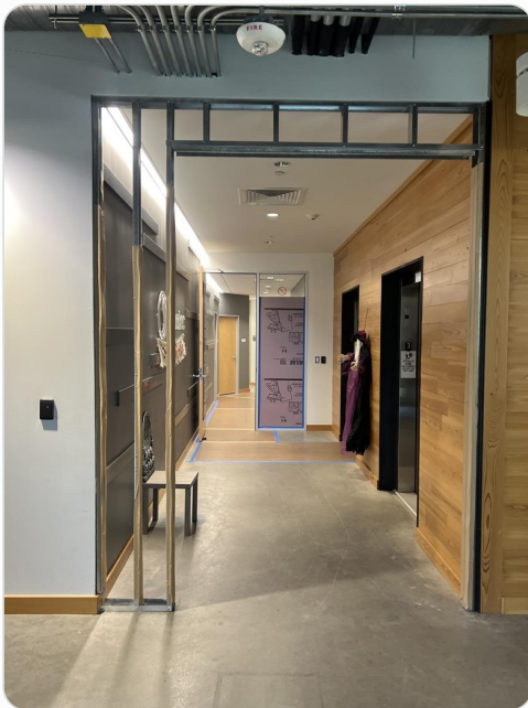
AUSTIN ENTRY ENCLOSURE IN PROGRESS
