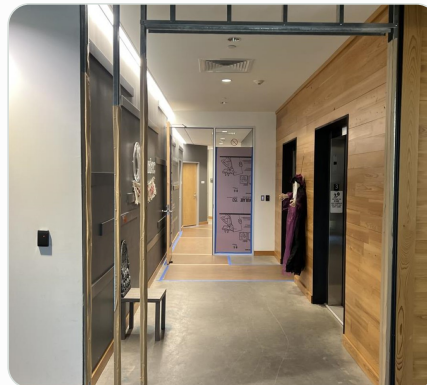
AUSTIN ENTRY ENCLOSURE IN PROGRESS
