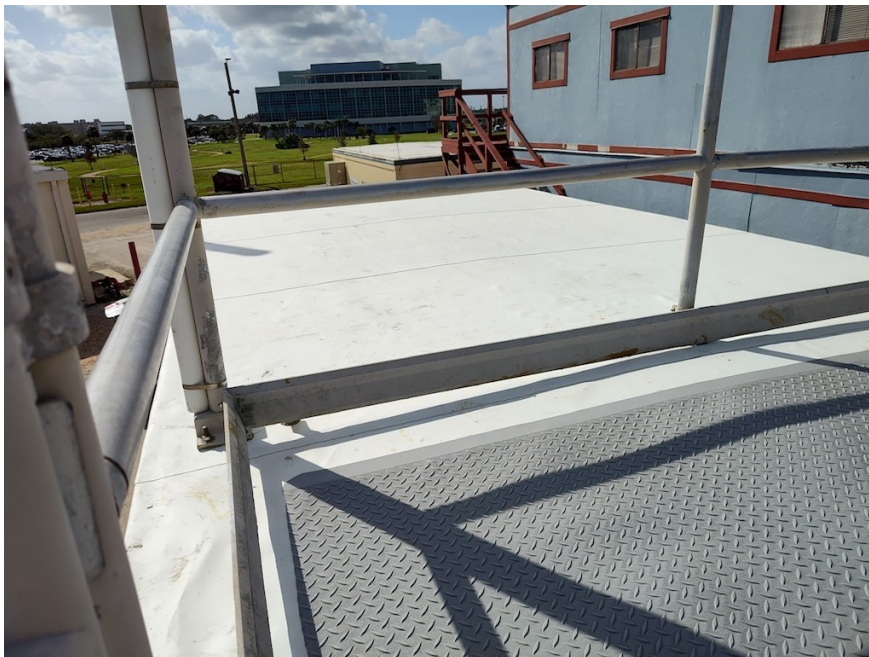
KENNEDY SPACE CENTER PRESS-SITE OFFICE | ROOF WORK
