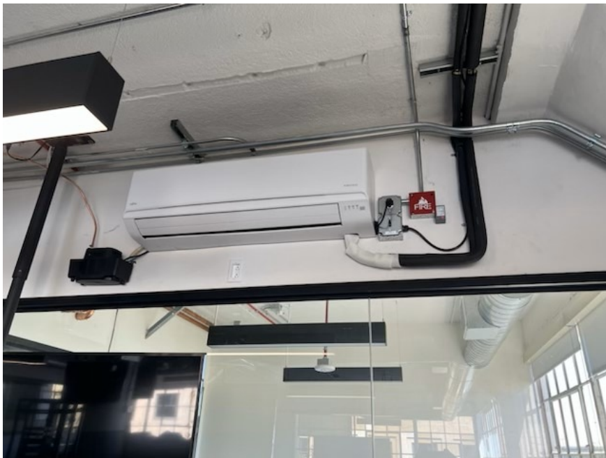
LOS ANGELES | HVAC AND OVERHEAD CONSTRUCTION
