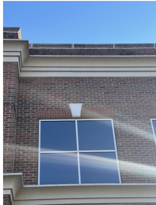
CHARLOTTE | EXTERIOR SIGNAGE REMOVED
