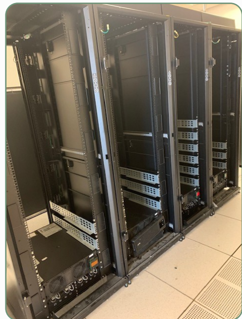
FLOOR 19 SERVER-SPACE TRANSITION | IN PROGRESS
