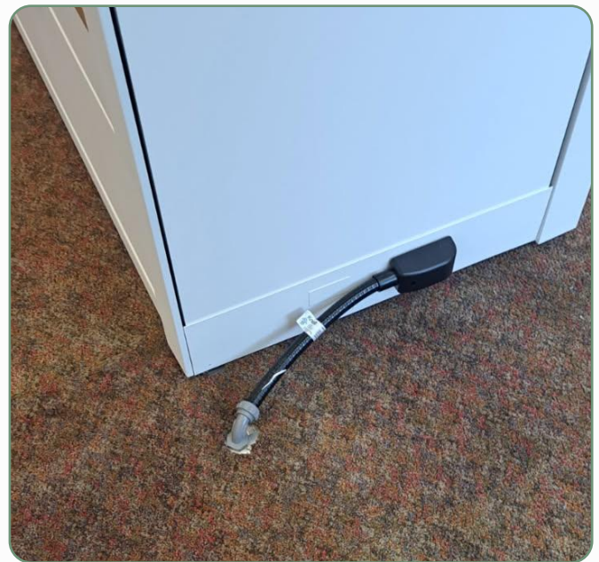
FURNITURE POWER RECONNECTION | COMPLETED
