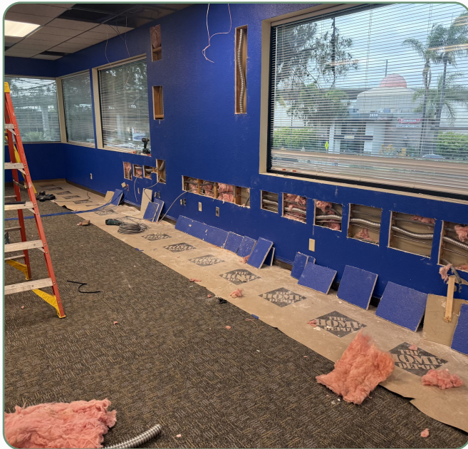
WALL OPENINGS FOR CIRCUIT RELOCATIONS | IN PROGRESS
