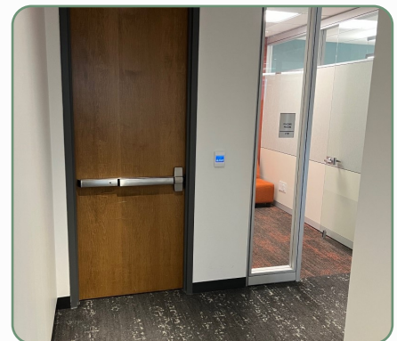
ENTRY AND PARTITION | COMPLETED
