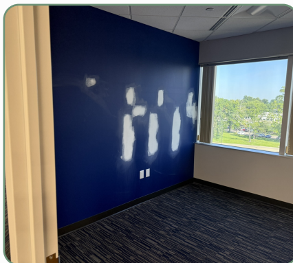
PAINT-READY REPAIRS | COMPLETED
