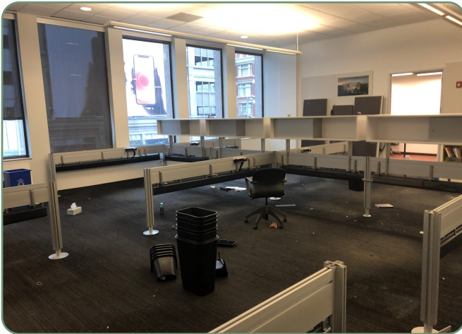
WORKSTATION DISMANTLING | IN PROGRESS
