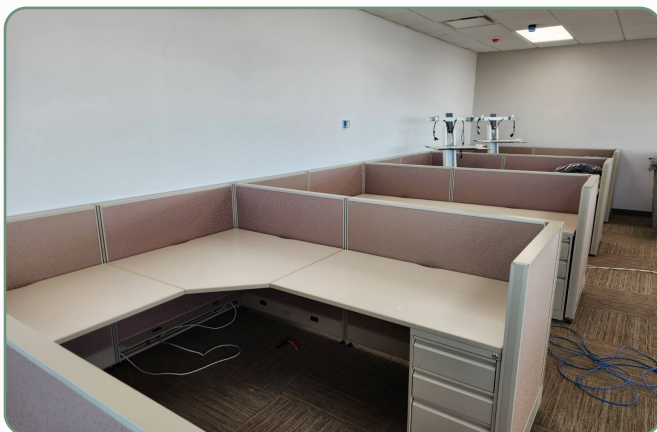
WORKSTATION INSTALLATION | IN PROGRESS
