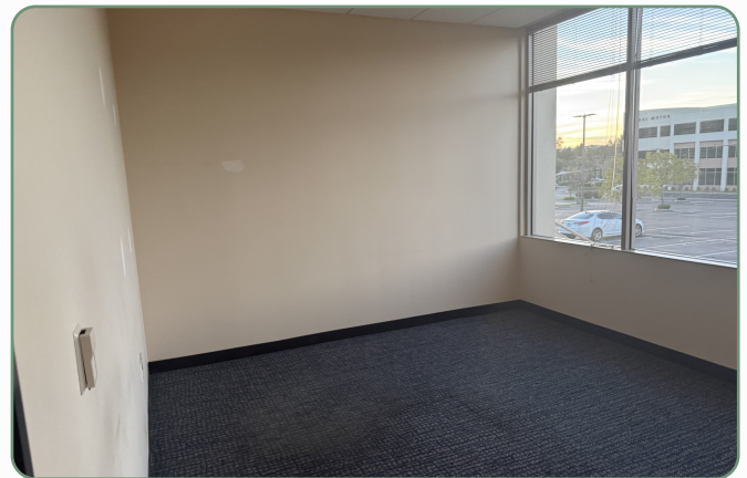
PRIVATE-OFFICE REMOVAL | COMPLETED
