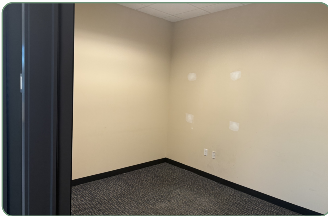
DRYWALL PATCHING | COMPLETED
