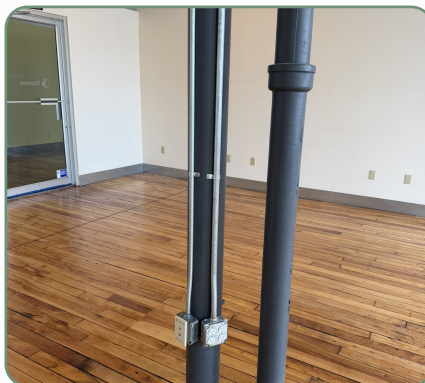
POWER INSTALLED | IN PROGRESS
