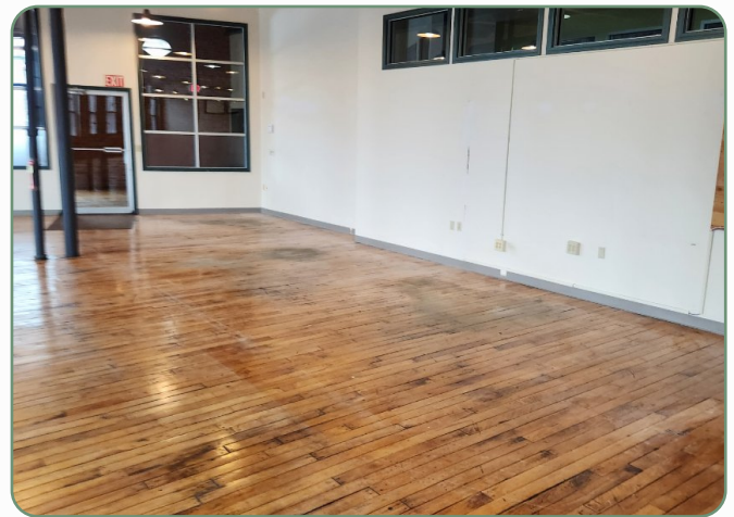
CLEARED OFFICE ZONE | COMPLETED
