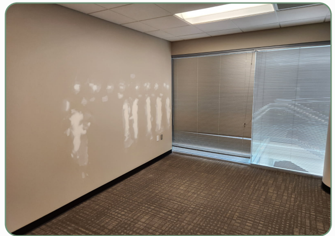
PAINT-READY WALL REPAIRS | COMPLETED
