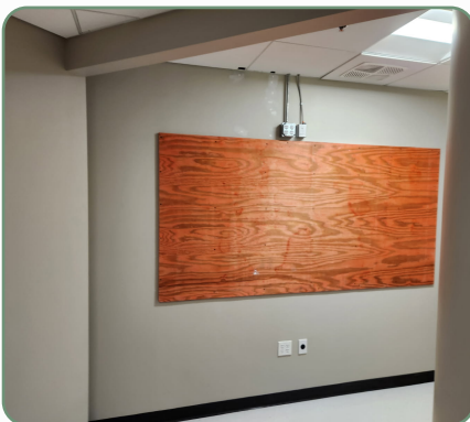
EQUIPMENT REMOVAL | COMPLETED
