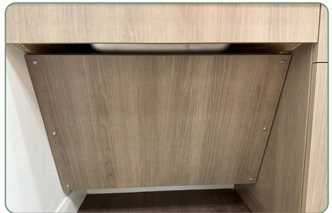
KNEE RECESS AND PANEL | COMPLETED
