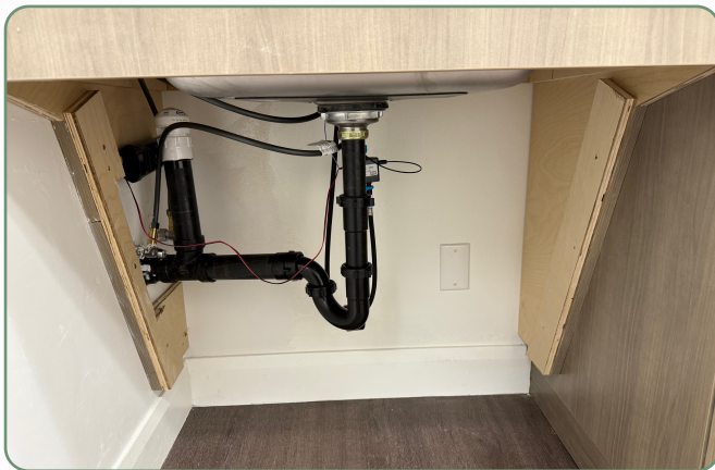
PLUMBING INTERFACE | IN PROGRESS
