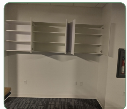
CLEARED CABINET SHELVEING | COMPLETED
