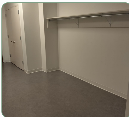
CLEARED STORAGE AREA | COMPLETED
