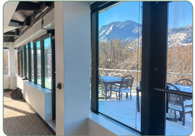
WINDOW-WALL FINISHES | IN PROGRESS
