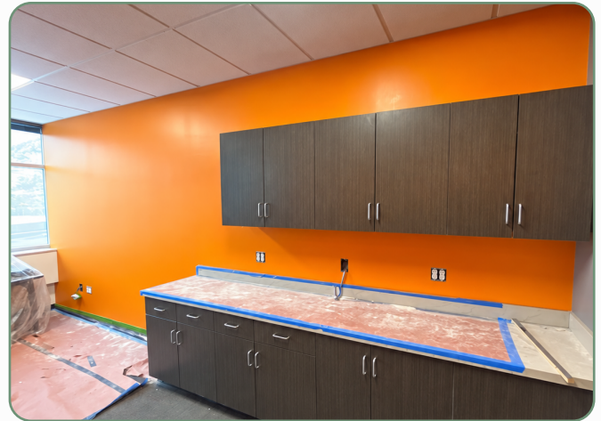
CABINET-AREA FINISHES | IN PROGRESS
